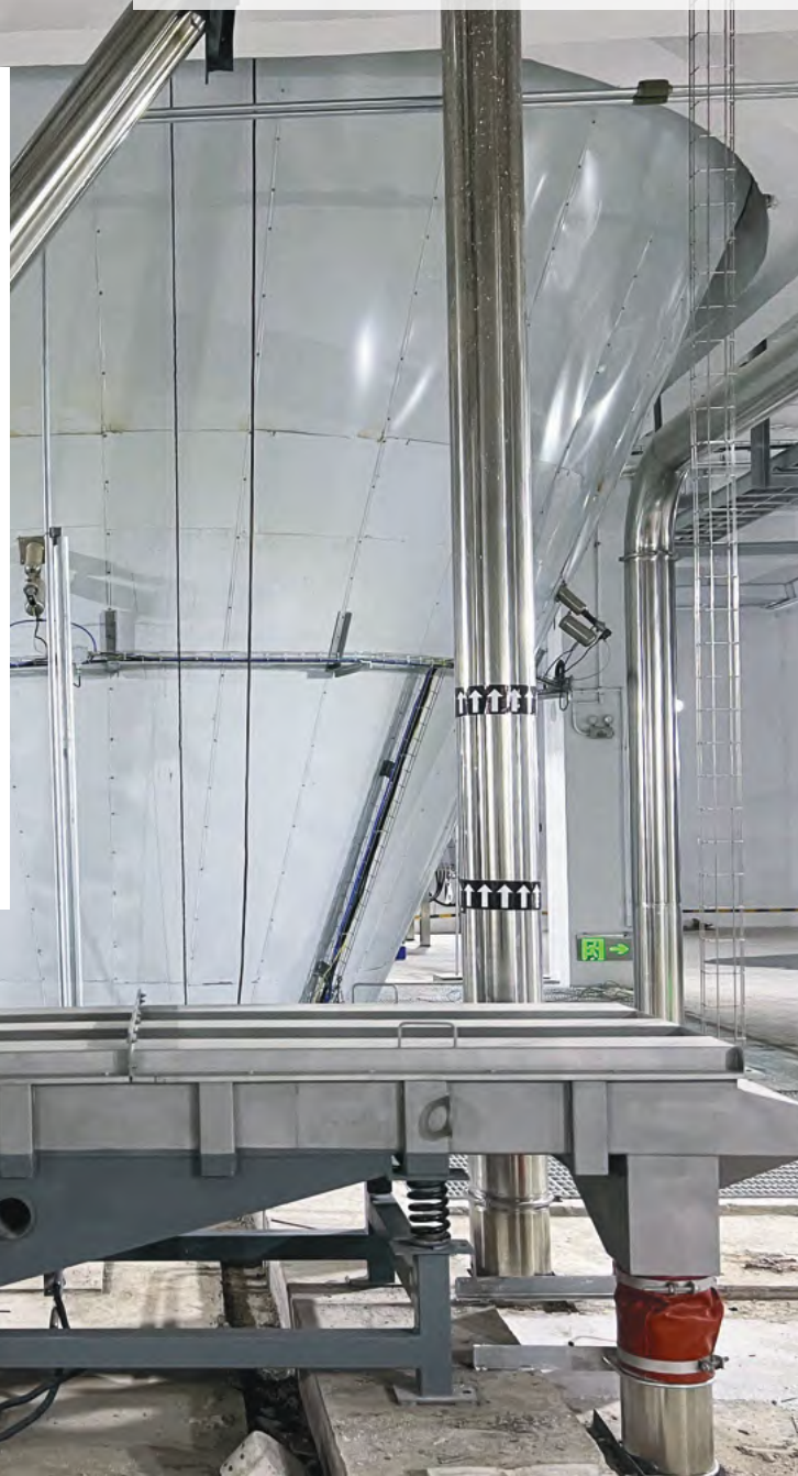
Drying tower & vibrating screen (Oriental Yuhong, 2017)
